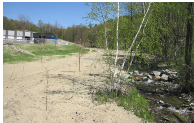
Figure 27. (Left) A berm blocked the floodplain of Beecher Hill Brook at the Hinesburg Town Garage. (Right) Floodplain restoration eliminated encroachments and restored a naturally functioning floodplain to establish a stable long-term channel. This project was funded by the Clean Water Initiative Program in partnership with the Lewis Creek Association.
