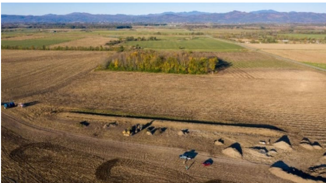
Figure 22. A wastewater disposal mound is a soil absorption system placed above the natural surface of the ground. The Town of Addison installed a community wastewater disposal mound system to treat municipal waste in June 2019. The project was financed by the Clean Water State Revolving fund.
